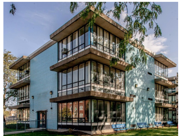
WPDG is redeveloping Overton Elementary School, a closed Chicago Public Schools facility, into 40 offices and a coworking space.
